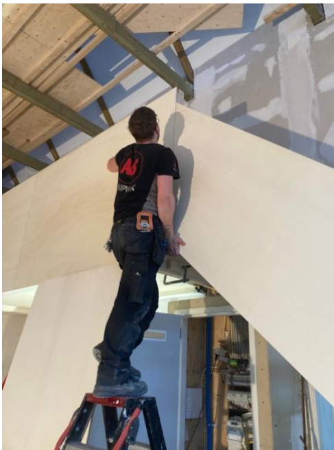
fitting the last panels by the stairs
